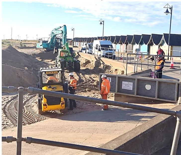
Unblocking the promenade drains near the Coral Café & the Seaholme Road pullover Photo: Trevor Wright 14th September
